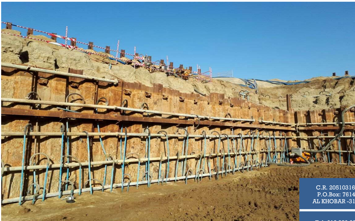
SSEM –DEWATERING & SHEET PILING @ SAUDI ARAMCO JAZAN KSA
