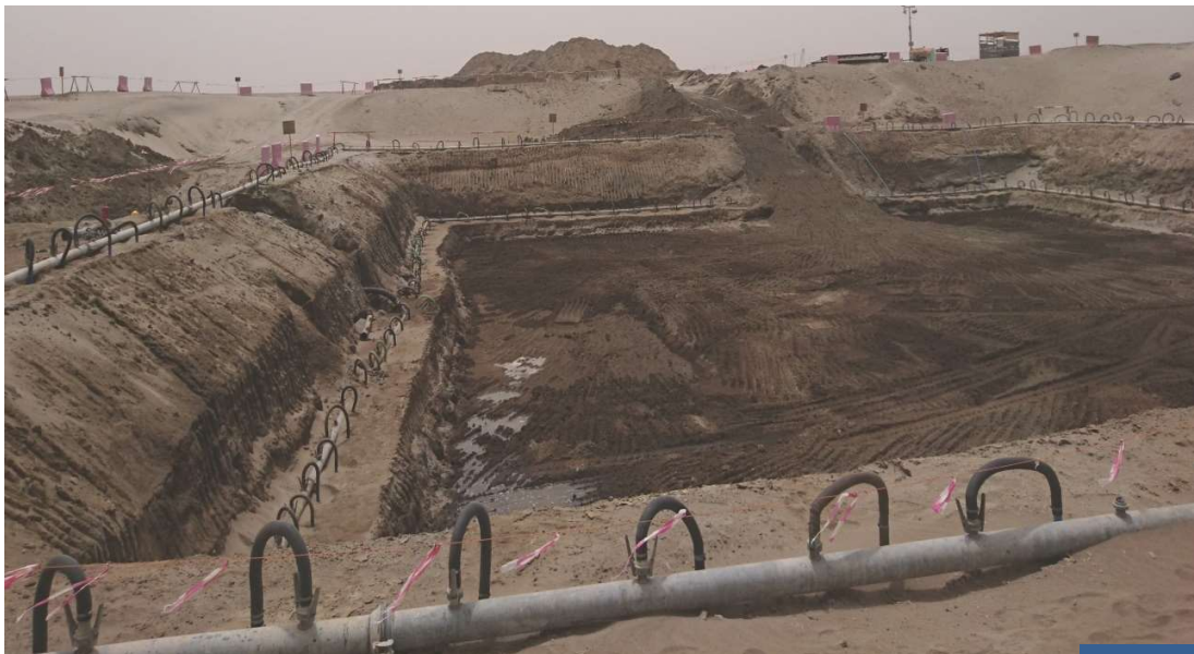
SSEM – JAZAN (RO/STP) PLANT – Dewatering & Sheet Piling Works
