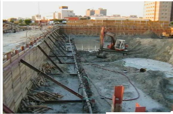
Dewatering works: For AL Nimer Bldg, Near Movenpick Hotel – Al Khobar.
