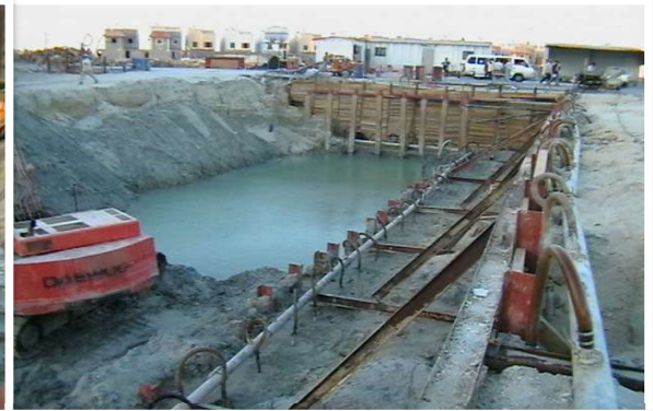
Dewatering works: For AL Nimer Bldg, Near Movenpick Hotel – Al Khobar.
