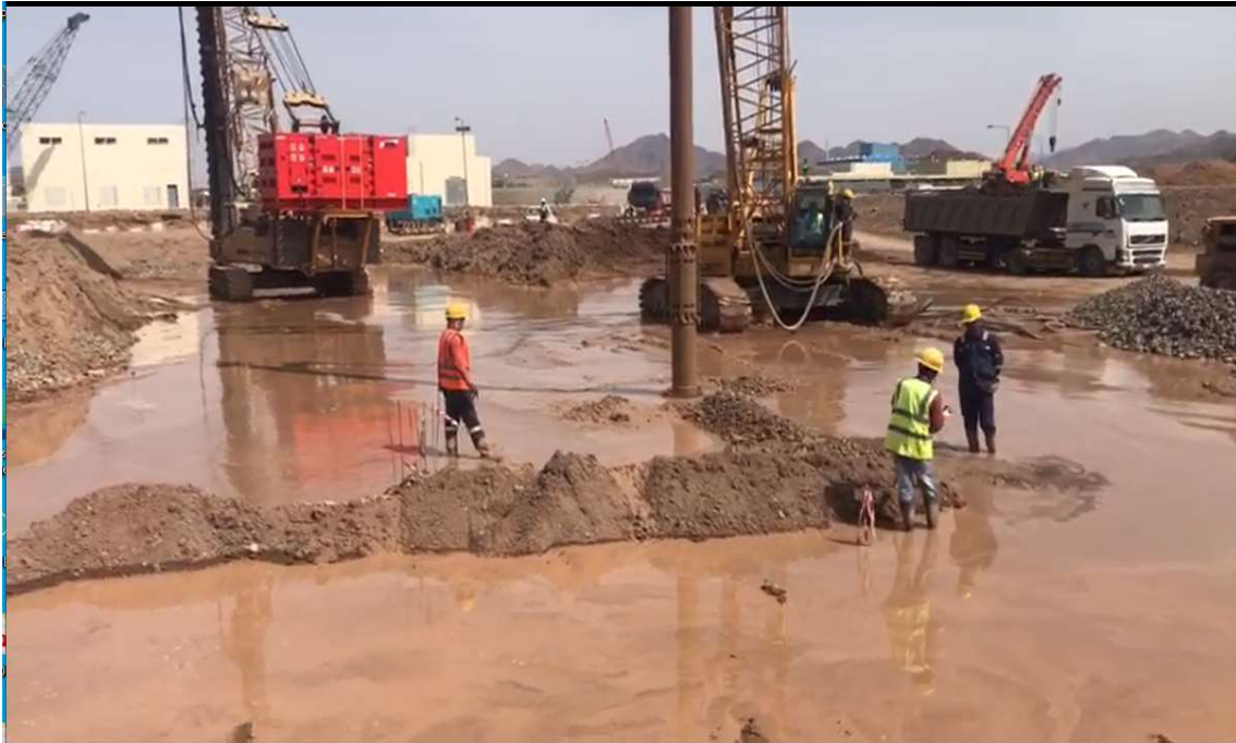
Soil Improvement (Stone Column) work For ISTP -3 PROJECT @ Madinah (Client ACCIONA JV TAWZEA, OWNER – SWCC)
