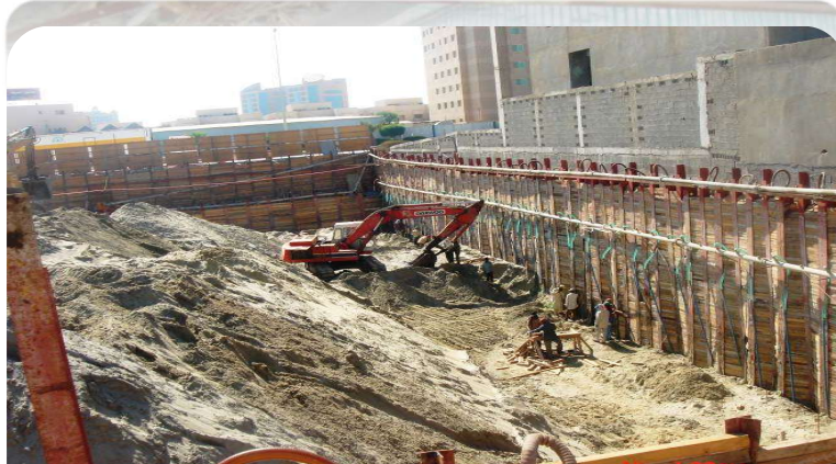
Shoring Works At Sheikh Abdullah Usman Tower
