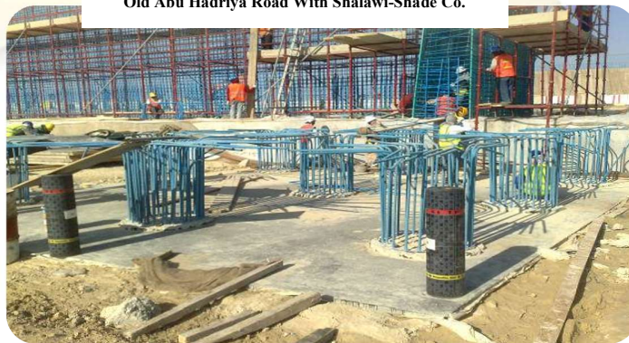
Concrete Piling For Bridge, Refinery Project Old Abu Hadriya Road With Shalawi-Shade Co.
