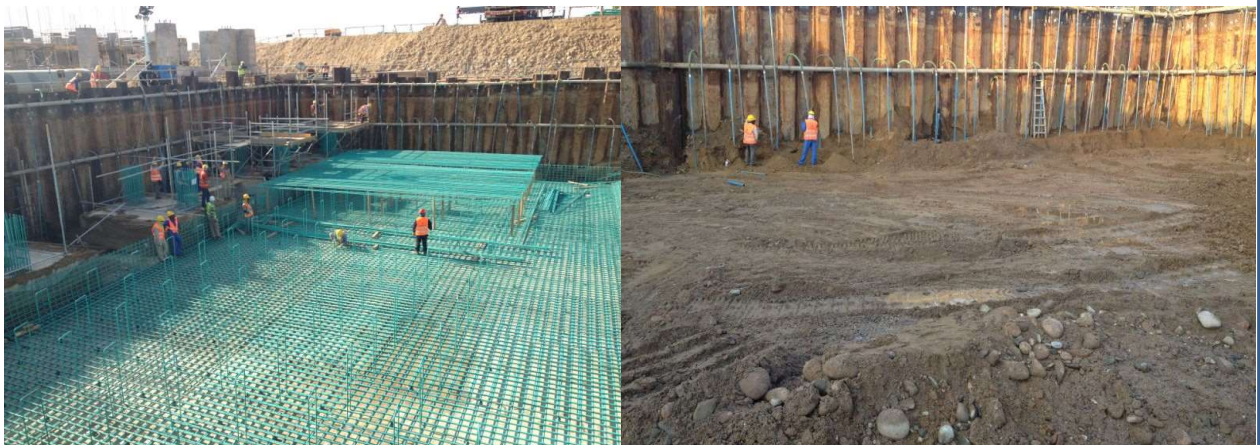
SHEET PILING WORKS FOR YERP PROJECT AT YANBU (CLIENT: SAUDI ARAMCO)
