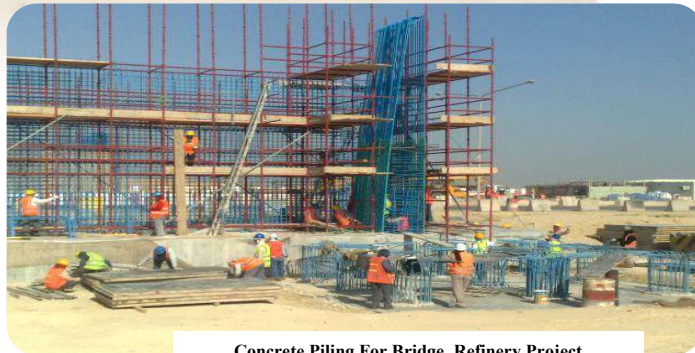
Concrete Piling For Bridge, Refinery Project Old Abu Hadriya Road With Shalawi-Shade Co.
