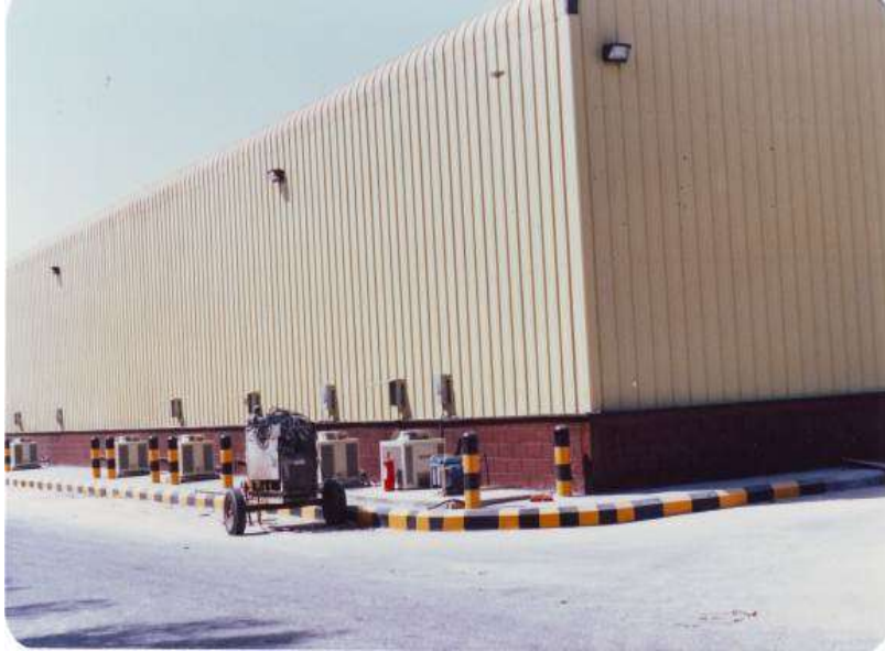
Mic-Procter & Gamble Ware House @ 2nd Industrial Area Dammam
