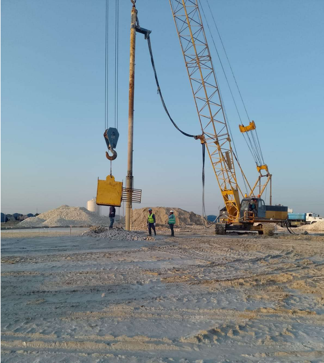
Soil Improvement (Stone Column) work For Contract No. 6510958281 @ WASIT JUBAIL KSA.
