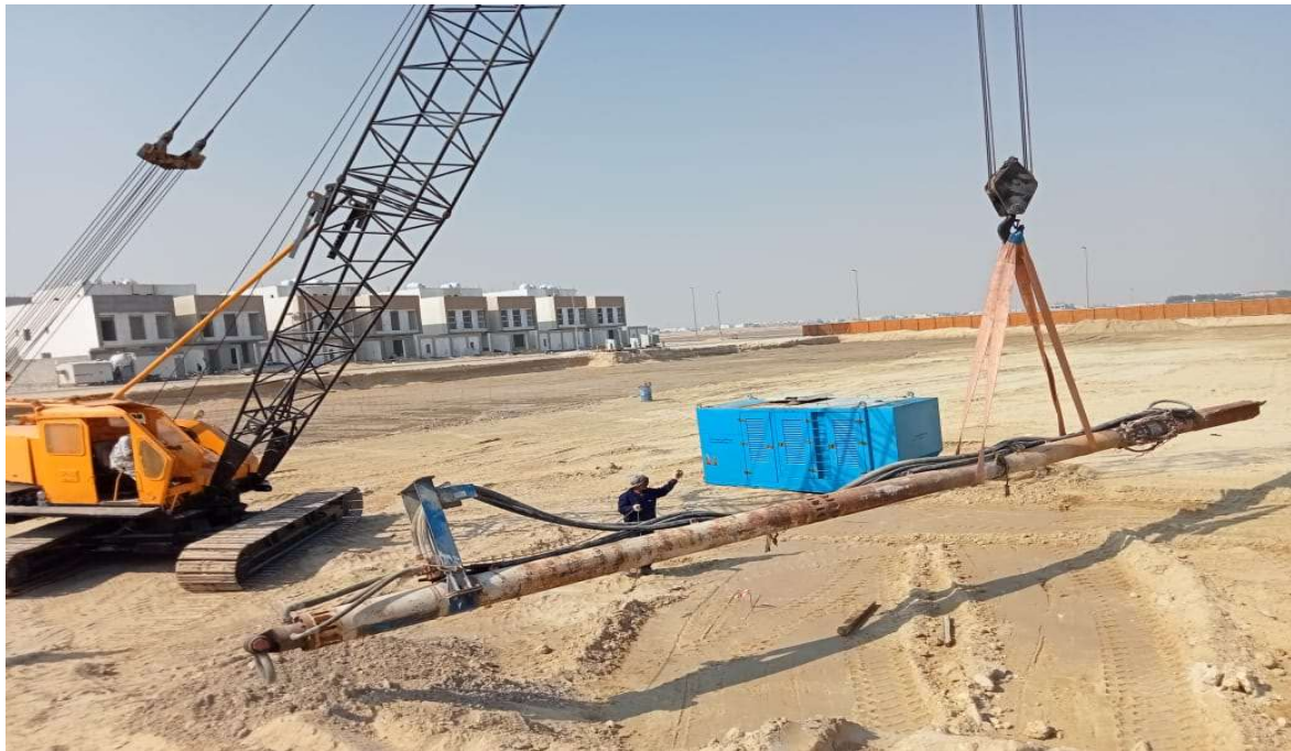
Soil Improvement (Stone Column) work For SWCC Project @ Al Khobar
