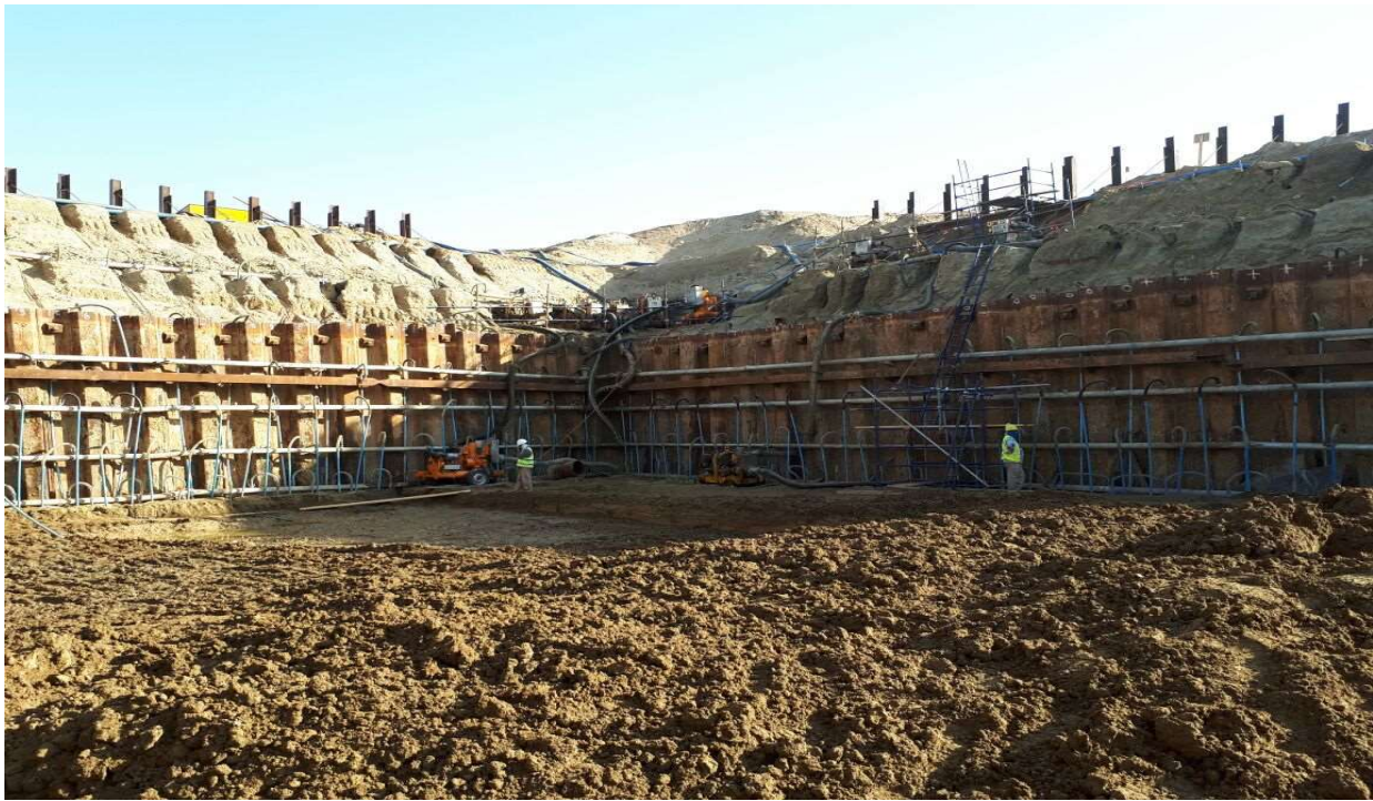
SSEM –DEWATERING & SHEET PILING @ SAUDI ARAMCO JAZAN KSA
